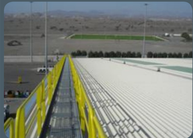
Testing facility in Casthouse
